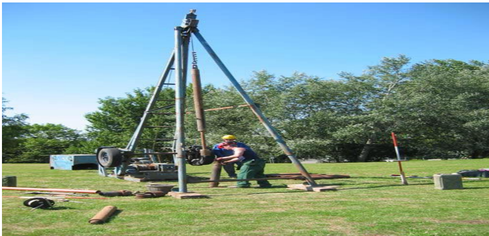
Fig 2: Shell and auger drilling
